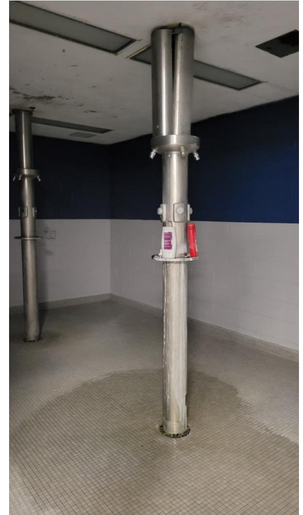
Leaking gang showers, worn ceilings in the locker rooms
