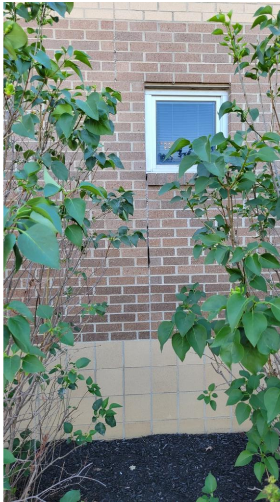
Failing caulk joint
