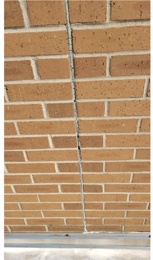
Failing Caulk Joint
