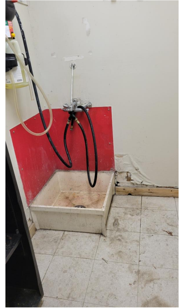
Gypsum board wall in not protected around the mop sink
