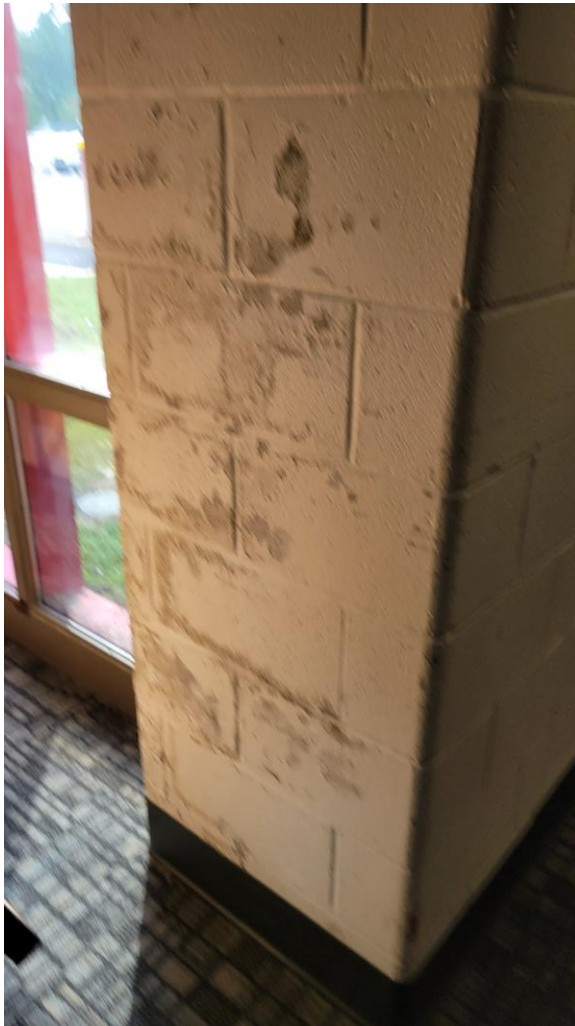
Moisture infiltration inside the building
