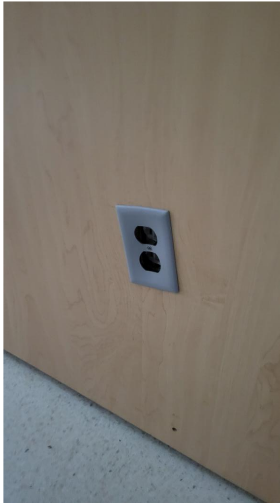
Plywood wall veneer is pulling away from the wall in the cafeteria (possible water infiltration from the courtyard)
