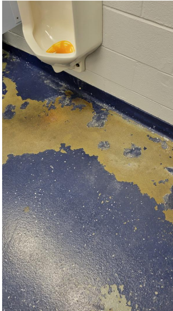
Worn epoxy flooring in wrestling locker room
