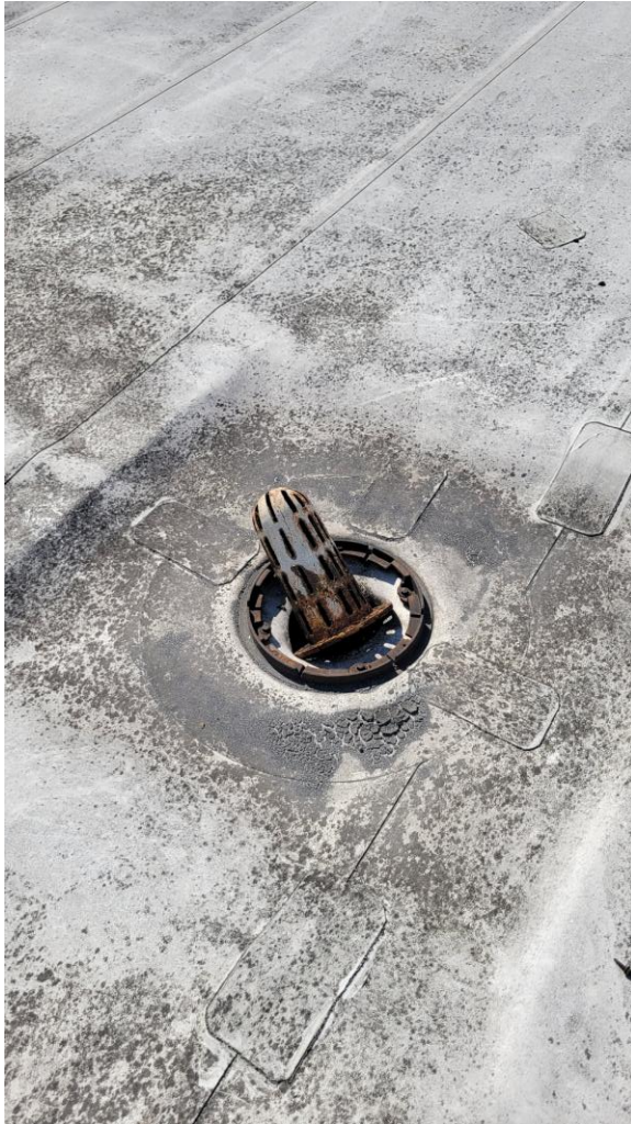
Single roof drain, no overflow
