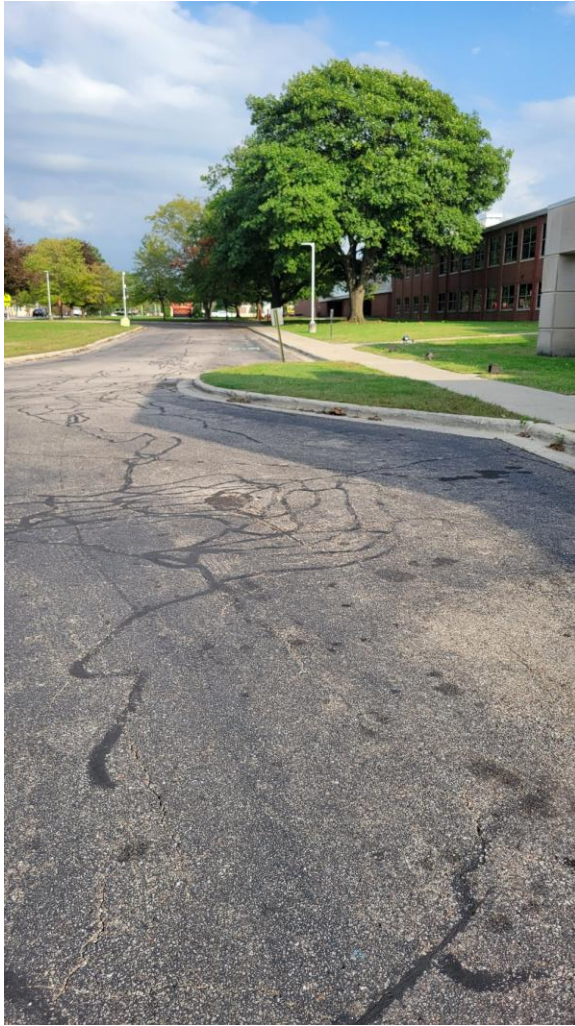
Cracking Asphalt on the north and east sides of the building
