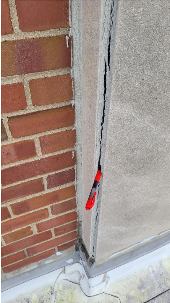
Failing caulk joint
