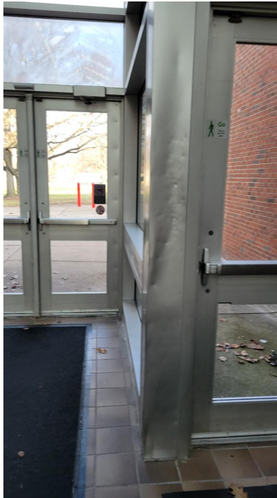
Damaged vestibule framing at pool entrance
