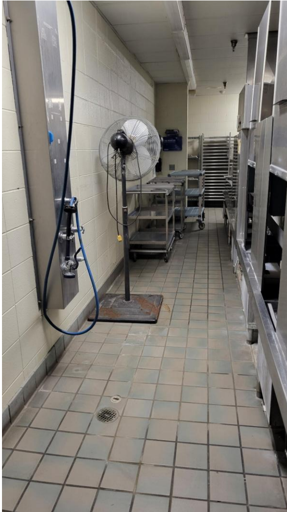
Fans in the dishwashing room. No air supply registers were observed during the site visit
