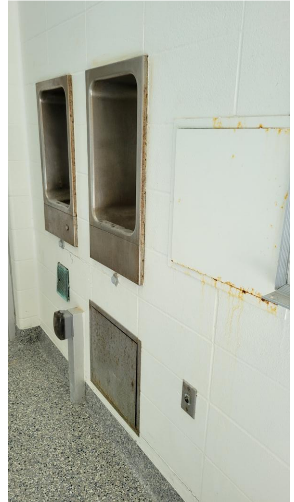
Rusting steel elements in the pool
