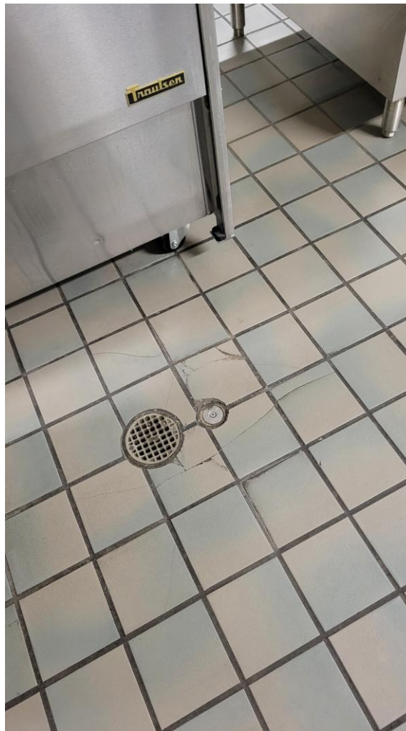
Cracked floor tile in the kitchen
