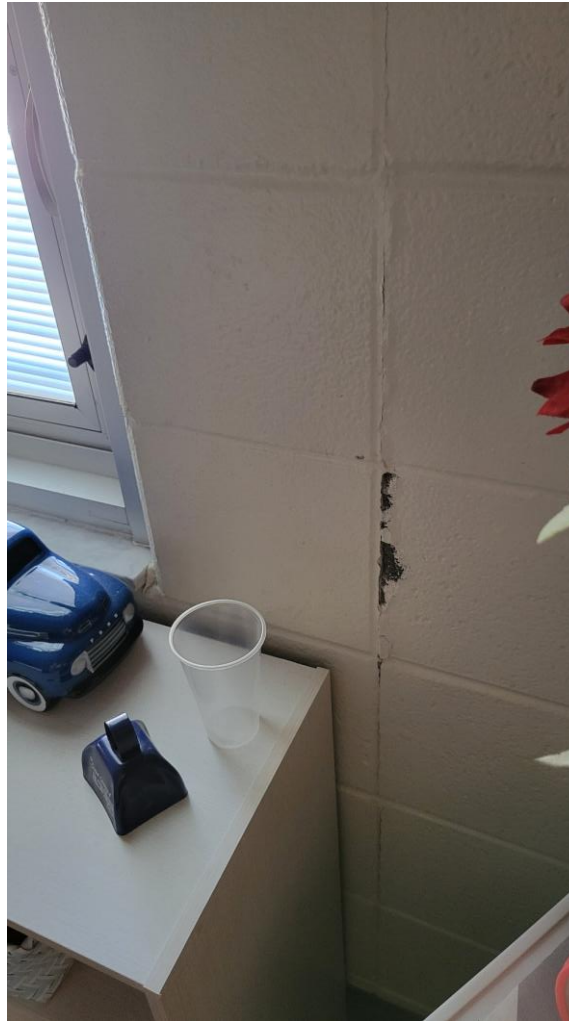
Moisture infiltration on exterior wall in classroom
