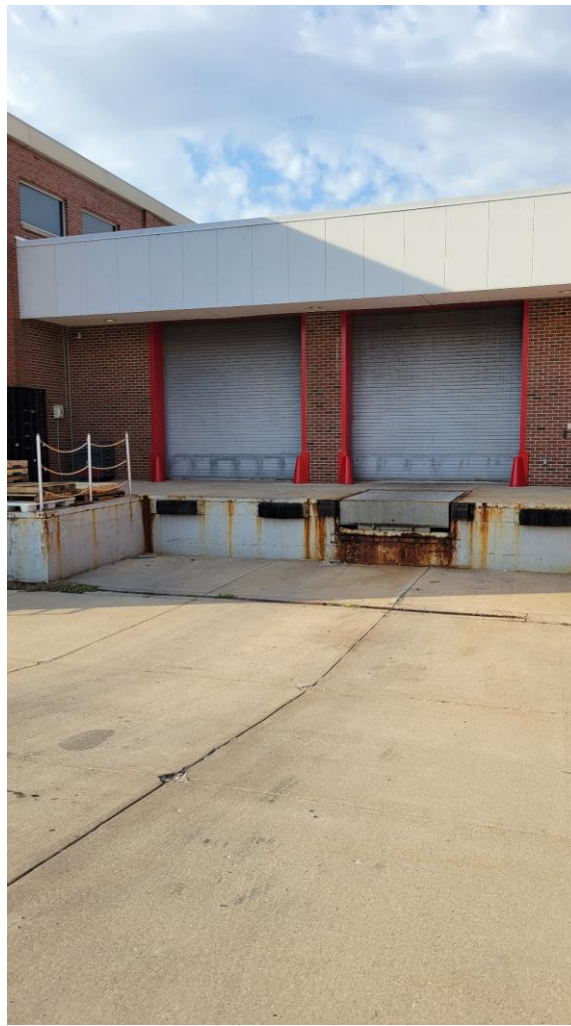
Rusting dock leveler and cracks in the concrete at the loading dock
