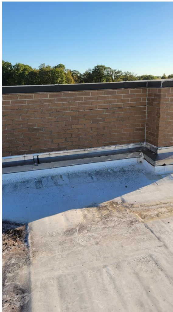
Loose mortar on parapet wall
