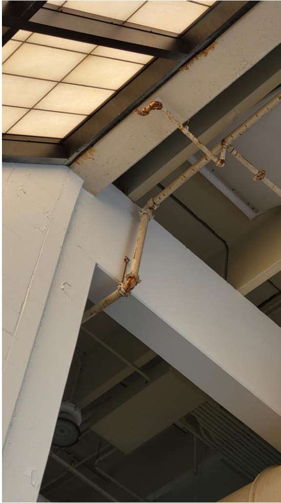
Pool rusting piping, peeling paint and yellowing skylight
