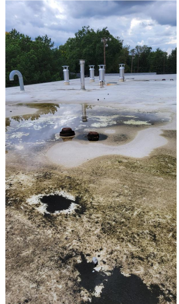
Ponding on the roof
